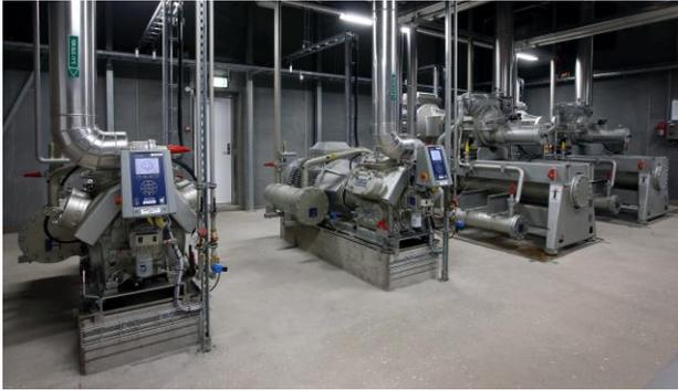
**Figure 2: Johnson Controls Heat pumps with UniSAB III controller.**
