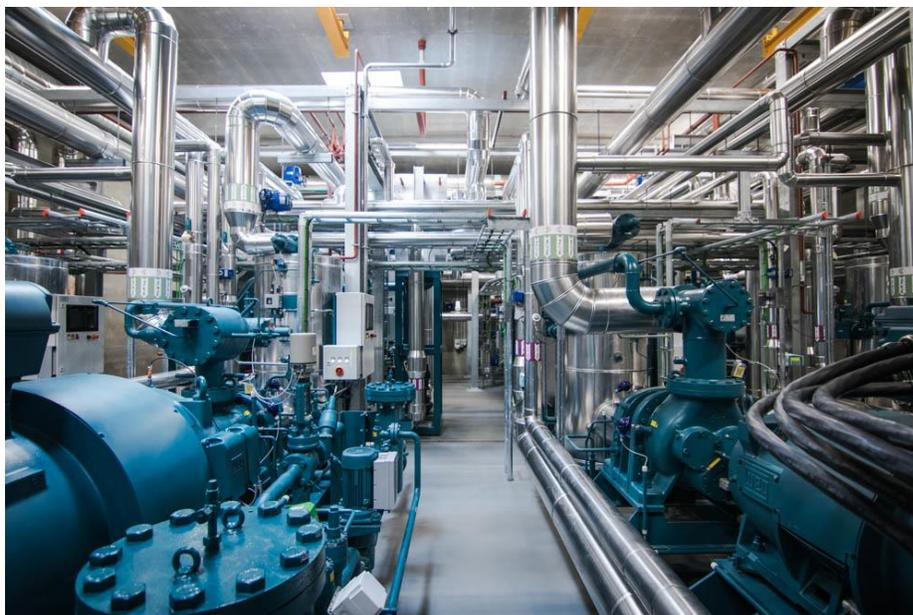
**Figure 1: 5 MW<sub>thermal</sub> heat pump system for district heating in Copenhagen [Source: HOFOR].**
